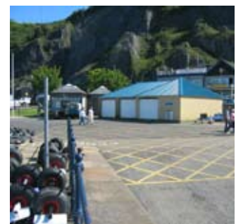
Existing facilities, Knab Rock
